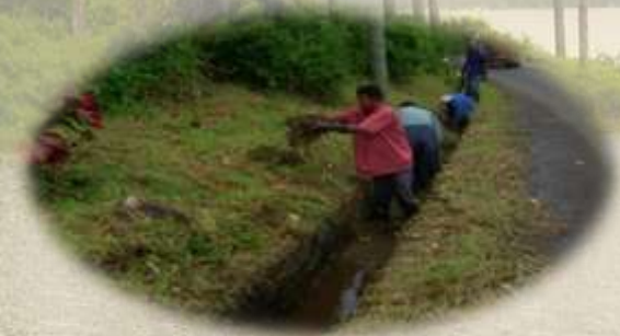
Cleaning of drains, canal rivulets and wastelands – clean ,green and safe town
